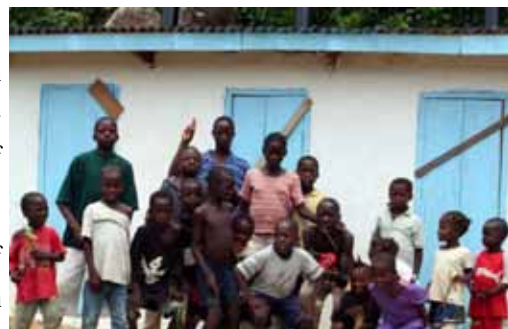
IRC School Latrine Block – Liberia May 2006
