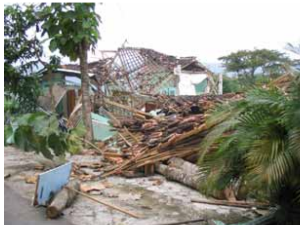
Debris post-earthquake. Bantul District, Java Island, May 2007
