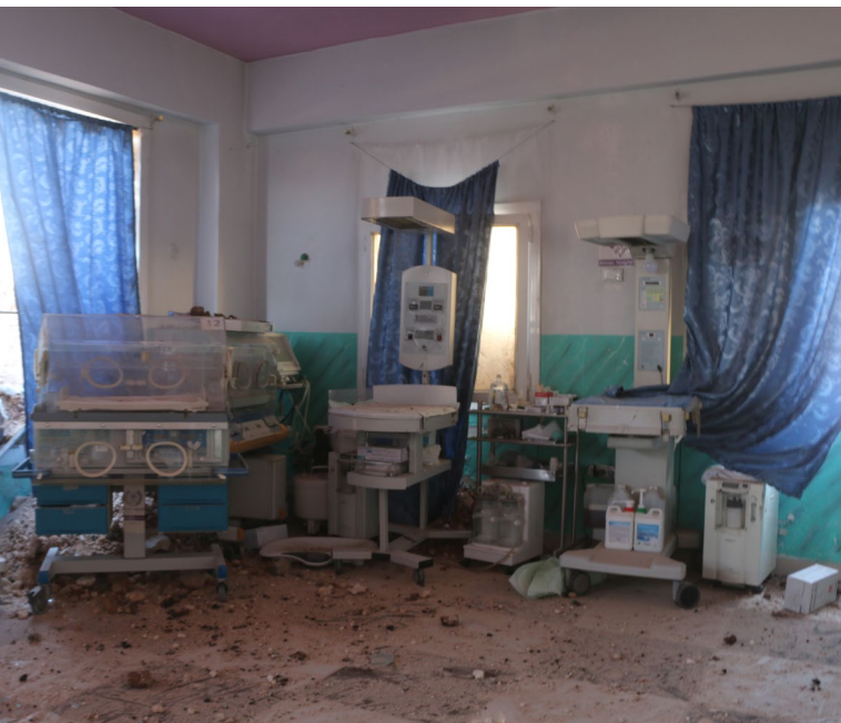
Eman hospital in Northwest Syria was targeted by airstrikes in 2019, completely destroying the building and leaving it out of service. PHOTO: frontlineinfocus
