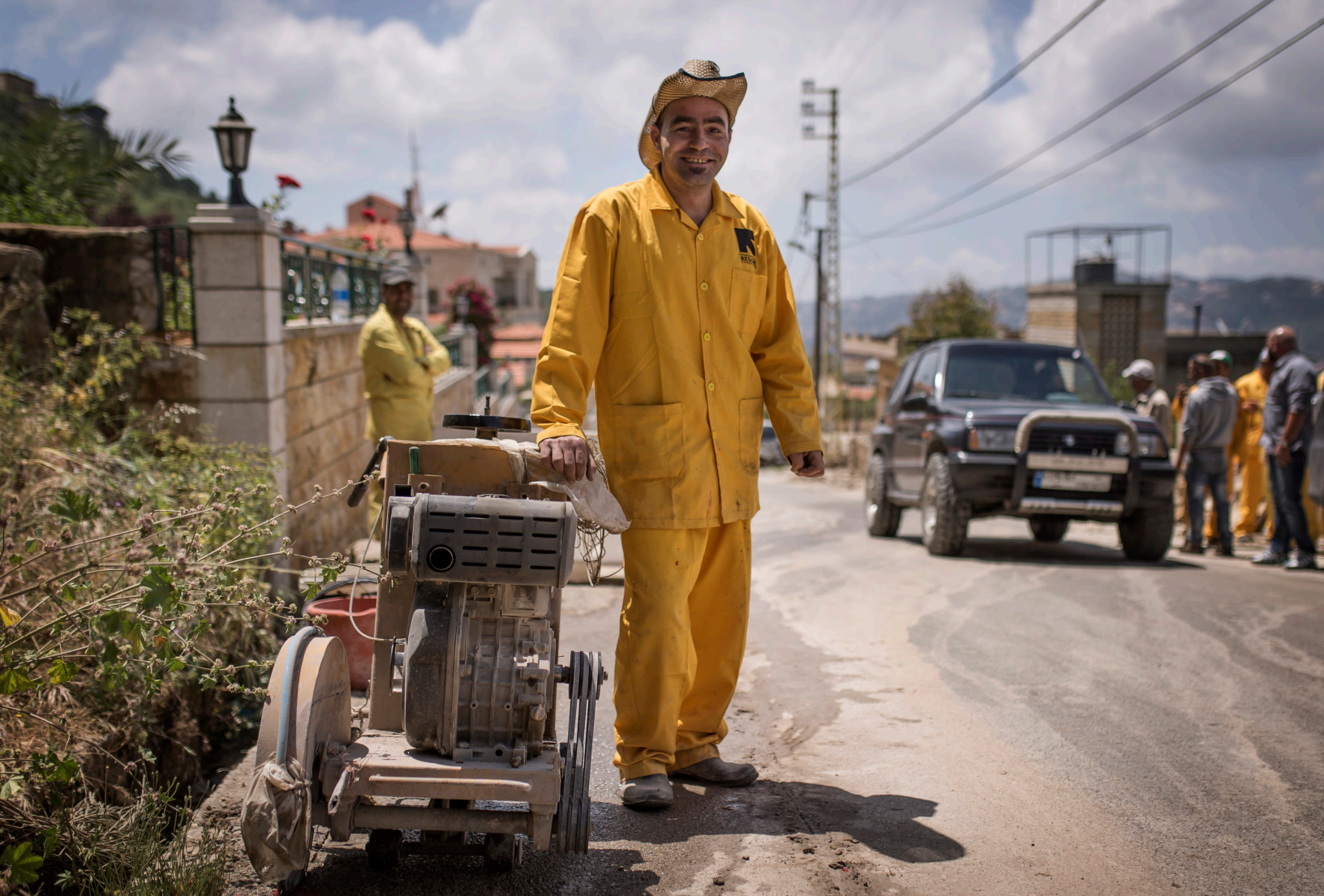
FRONT: ANNIE GRANT, 27, RUNS A STALL AT IN THE MONROVIA SUBURB OF PIPELINE. "I MAKE ENOUGH MONEY NOW TO SEND MY CHILDREN TO SCHOOL," SHE SAYS. PETER BIRO/IRC BACK: SYRIAN REFUGEES IN AN IRC CASH-FOR-WORK PROJECT LAY SEWAGE PIPES IN SALIMA, MOUNT LEBANON JACOB RUSSELL/IRC
