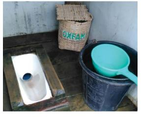
Figure 3: A design for a lined bin attached to the wall (Oxfam-Nepal, 2015). Note, it must also be easy to empty to prevent the cleaner from handing pads directly.
