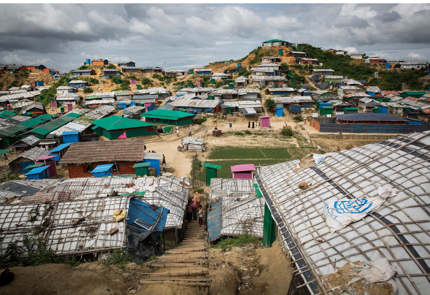
The Rohingya camps in Teknaf and Ukhiya were constructed by cutting down hills, with shelters resting on loose, sandy land. Photo from 2018 by Ingebjørg Kårstad/ Norwegian Refugee Council.
