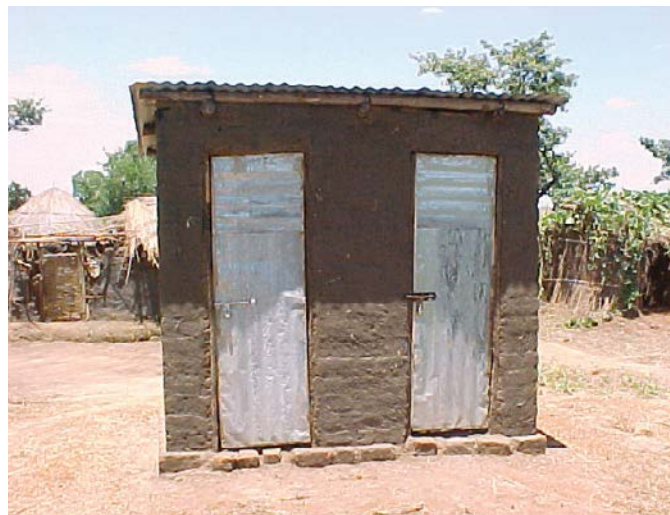
Toilets in a refugee camp in Northern Uganda. IRC
