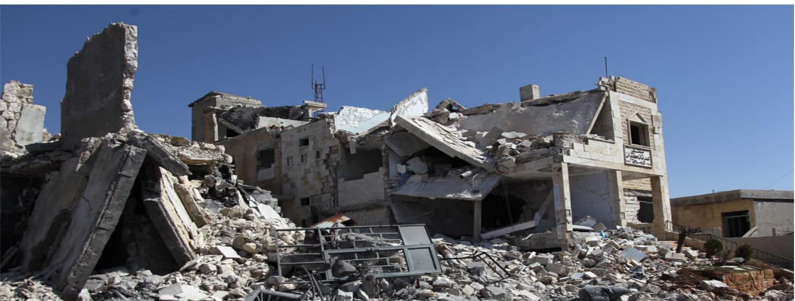
Damage caused by an airstrike to Kiwan Charitable Hospital, supported by IRC's partner organization, SEMA in northwest Syria. Credit: frontlineinfocus
